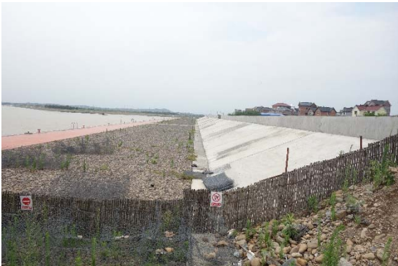
左岸上游防洪堤 (2016.6)
