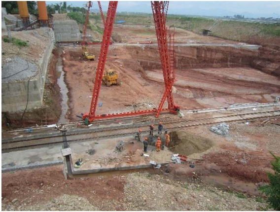
电站厂房基坑开挖 (2013.6)
