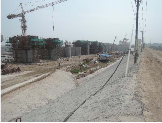
左侧泄洪闸施工 (2016.3)
