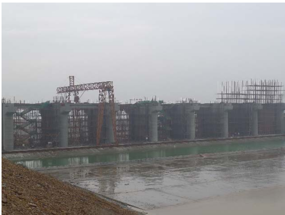
右侧泄洪闸施工 (2014.6)
