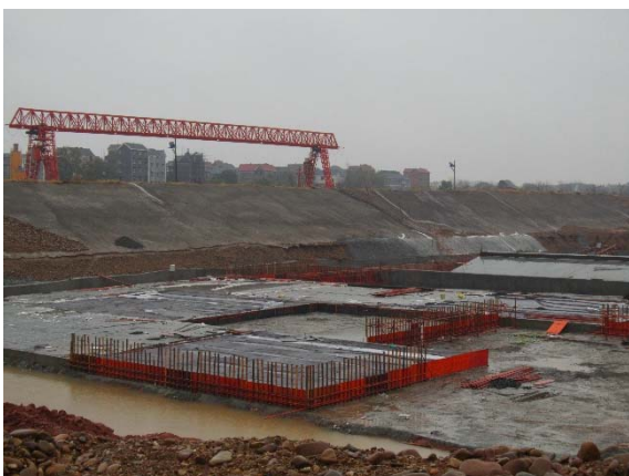
围堰喷砂护坡 (2013.12)
