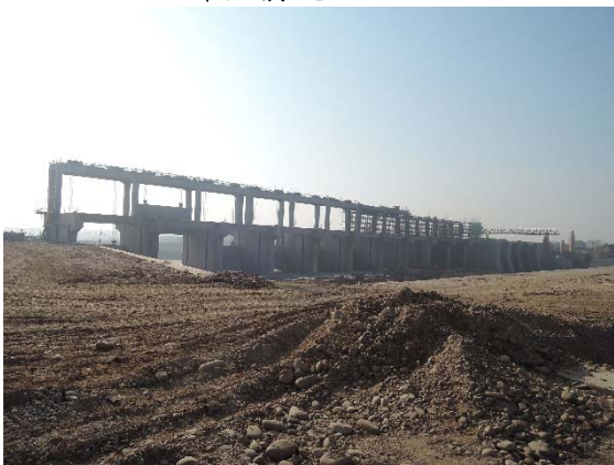
电站厂房及右侧泄洪闸施工 (2014.11)
